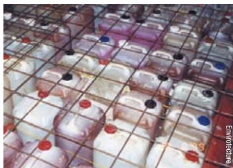
These void formers are mostly expanded foam boxes, which interfere with earth coupling, but more thermally connective alternatives are available. These include proprietary systems that use recycled tyres, or re-used detergent bottles filled with water and grouped together as void formers.
