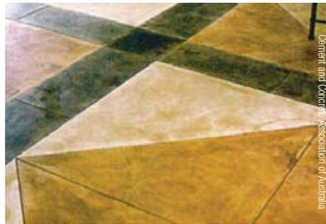
Coloured concrete can be used in either steel trowel or burnished finishes, to achieve various results. It may be advisable to use experienced specialist contractors to carry out this work. These can be applied as oxides in the mix, or as 'dry shake' pigments applied to freshly screeded concrete and then trowelled in, or by chemically staining the concrete.
