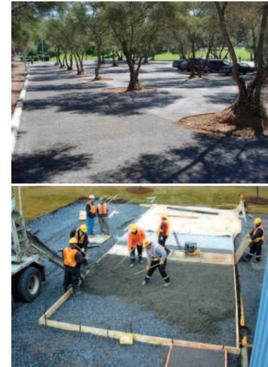
because the pavement itself acts as a retention area. Parking lot owners will spend fewer dollars on labour, construction and maintenance of retention ponds, skimmers, pumps, drainage pipes and other stormwater management systems. Expensive irrigation systems can also be downsized or eliminated. A pervious concrete parking lot will help reduce demands upon sewer systems.
