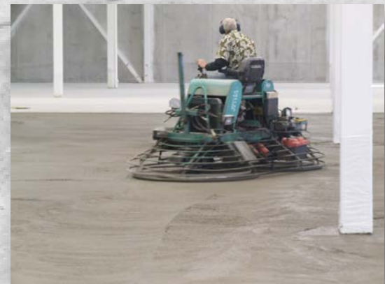
Ride on power trowel
