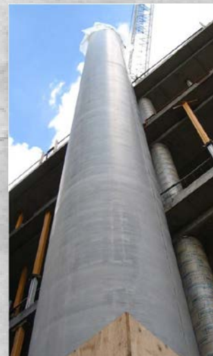
Self Consolidating Concrete (SCC) significantly reduces bugholes and can be used in architectural concrete applications
