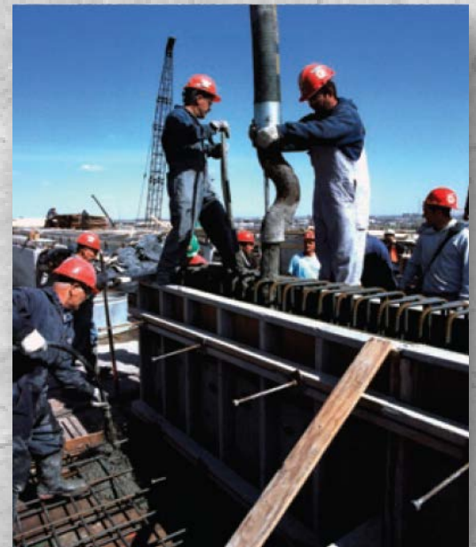
Concrete pumping on a commercial project using a flow restriction device to provide resistance to flow and to prevent direct free fall
