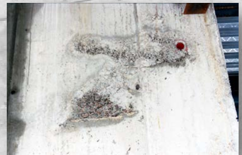
Honeycombing in a concrete column
