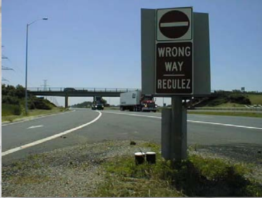
Concrete cylinders used for concrete acceptance purposes must be stored in a temperature controlled environment - not left to bake in the sun
