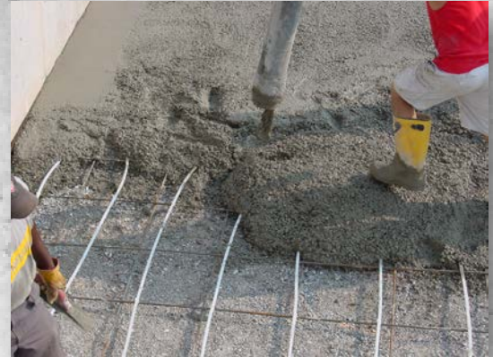
Concrete pumping on a residential radiant floorheating project
