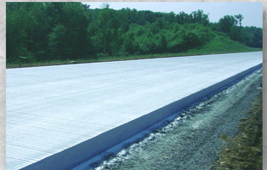
The proper application of a curing compound
